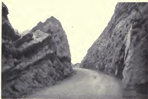
Cutting on the road near the Mumbles
